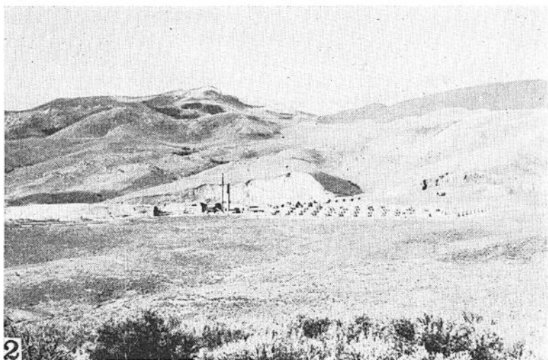
FIG. 2. Getchell Mine, Nevada. The scars on the hill behind the camp mark the footwalls of the open pits.
