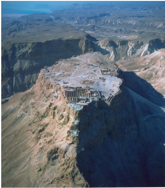
Figure 4 This view of the reconstructed storerooms of Masada shows the long, unsupported walls that are susceptible to earthquake damage.
