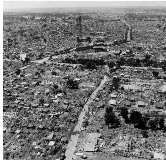
Figure 12 Photo showing nearly complete devastation in the Lunan district of the city of Tangshan from the 1976 Tangshan, China, earthquake (Huixian et al. , 2002). Tangshan was a major industrial center with a population of 1 million before the earthquake, which occurred directly under the city at 3.42 a.m. About 93% of residential buildings and 78% of commercial buildings in the city were destroyed (Yong et al. , 1988). The officially reported death toll is 255 000, but estimates are as high as 655 000. Reproduced with Housner GW, Lili X, and Duxin H (2002), with permission.
