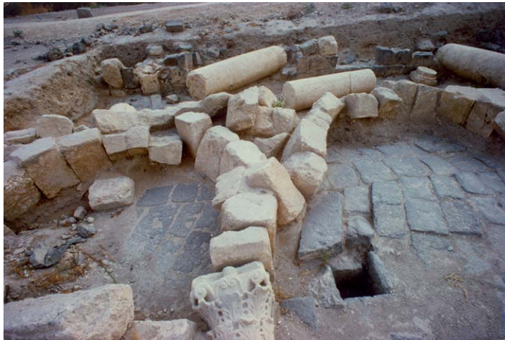
Figure 7 These arches are from Bet Shean, 45 km south of Susita, shown in Figure 6 . These arches collapsed out into the street, probably in the same earthquake as destroyed Susita in AD 749.
