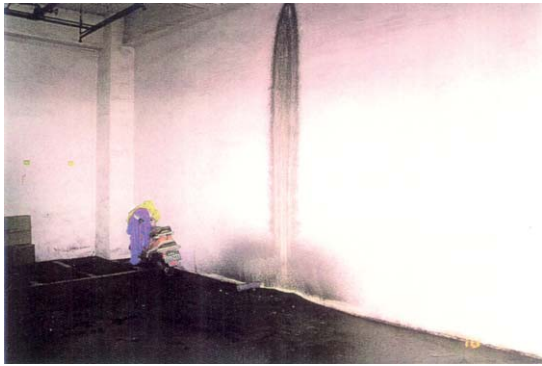
Figure 1 Smear left on a building wall created by ejected sand during the 1999 M 7.5 Chi-Chi earthquake in Taiwan. Motorcycle at lower left shows scale. Reproduced from Su T-C, Chiang K-W, Lin S-J, Wang F-G, and Duann S-W (2000) Field reconnaissance and preliminary assessment of liquefaction in Yuan-Lin area. Sino-Geotechnics 77: 29–38.
