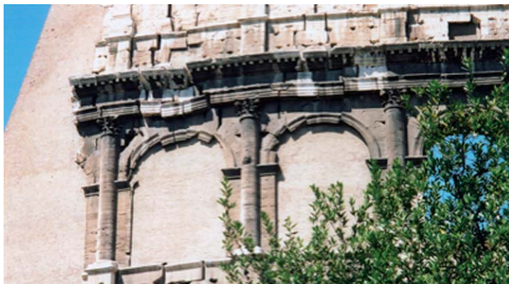
Figure 9 These arches are from the outer wall of the Colosseum in Rome. Once, there were more arches to the left of the leftmost one in this photo, but they collapsed in an earthquake. Note the chaotic state of the keystones in the leftmost remaining arch.
