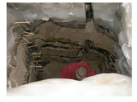
**Subglacial Processes, Figure 2** A 4.5 m thick excavation in deforming subglacial permafrost beneath Wright Lower Glacier in the McMurdo Dry Valleys, Antarctica. Measurements over 3 years demonstrate that deformation extends more than 3.5 m beneath the ice-permafrost boundary and that most deformation is accommodated by ice-rich layers between frozen sediment layers. The bolts and stakes have been used to measure strain and velocity over a period of 4 years.
