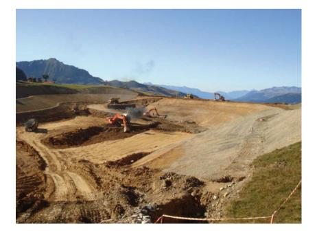
Artificial Production of Snow, Figure 4 Water storage reservoir being built for artificial snow production (Photo: Benjamin Damelet).
