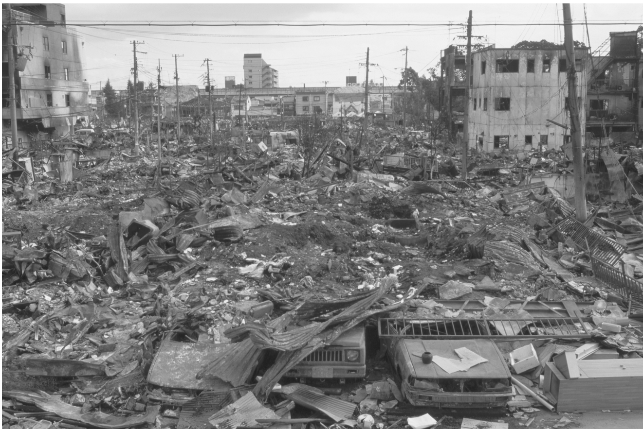
FIGURE 8.35 Damage from the Kobe earthquake in 1995 (Japan).
