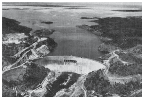
Fig. 240 The Kariba Dam across the Zambezi River with a high of 175m and holding back one of the largest artificial lakes in the world. It lies between Zimbabwe on the right side and Zambia on the left (1964)
