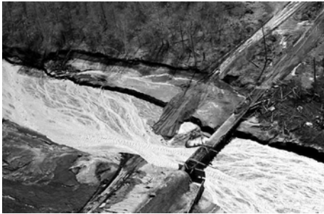
Fig.5. The road and the dam in the area of river Bekesh were destroyed with mud flows. Photo by Yu.V. Demyanchuk.
