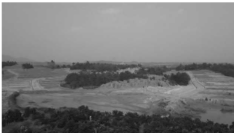
Figure 3.5 Soil pollution due to rare earth mining in Jiangxi Province
