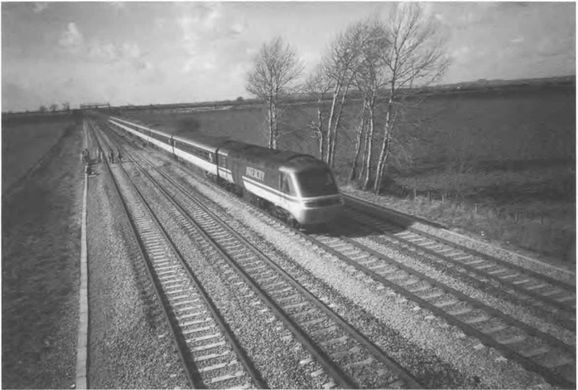
FIG. 10.1. (b) Railway embankment. Poor compaction and steep slopes are characteristic of this type of embankment (Perry et al. 2003).
