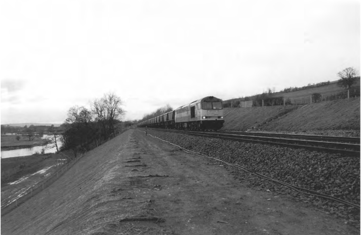
FIG. 10.3. An example of construction on side-long ground; in this case a railway with tracks supported on a repaired slope failure.
