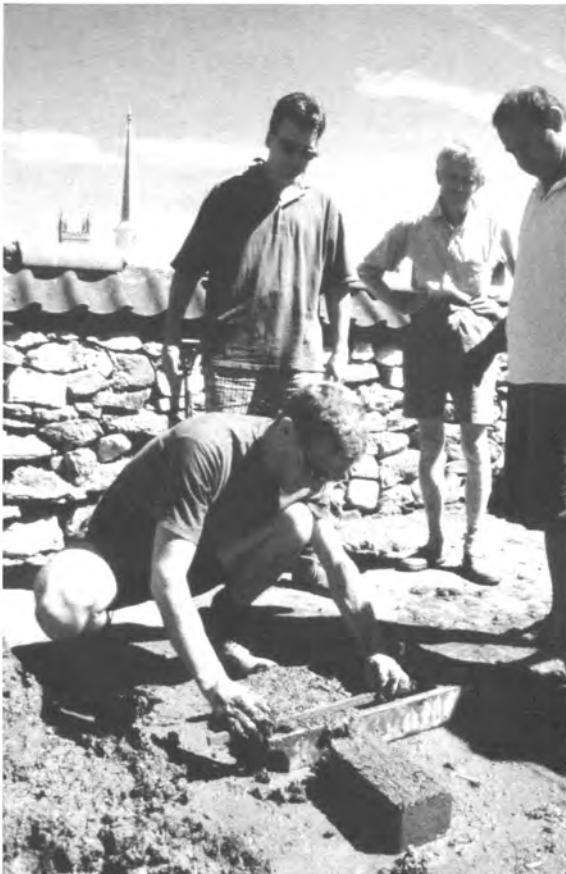
FIG. 13.4. The manufacture of adobe blocks by University of Plymouth Students.
