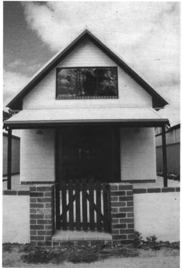
FIG. 13.2. Speculative housing at Margaret River, Western Australia (1997).
