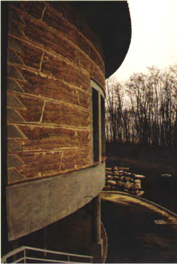
PLATE 5. New church at Anse, near Lyon, France.
