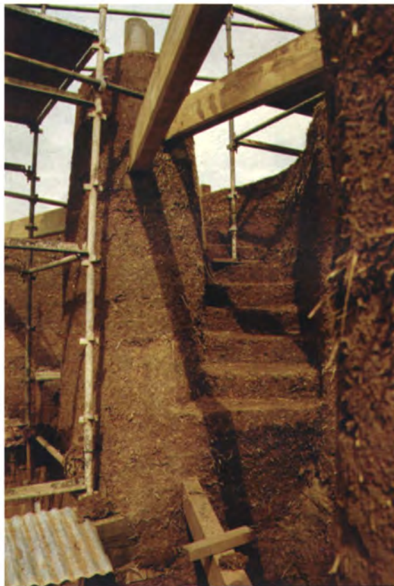
PLATE 12. Keppel Gate cob house under construction, Ottery St. Mary, East Devon.
