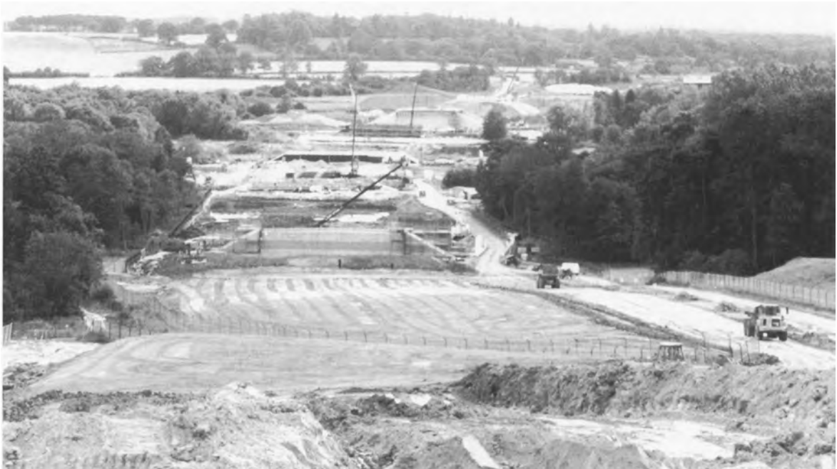
FIG. 10.21. A34 Newbury Bypass. Construction across soft ground, dewatered to allow use of clay fill. The works involved a series of bays with due consideration of surrounding wetlands.
