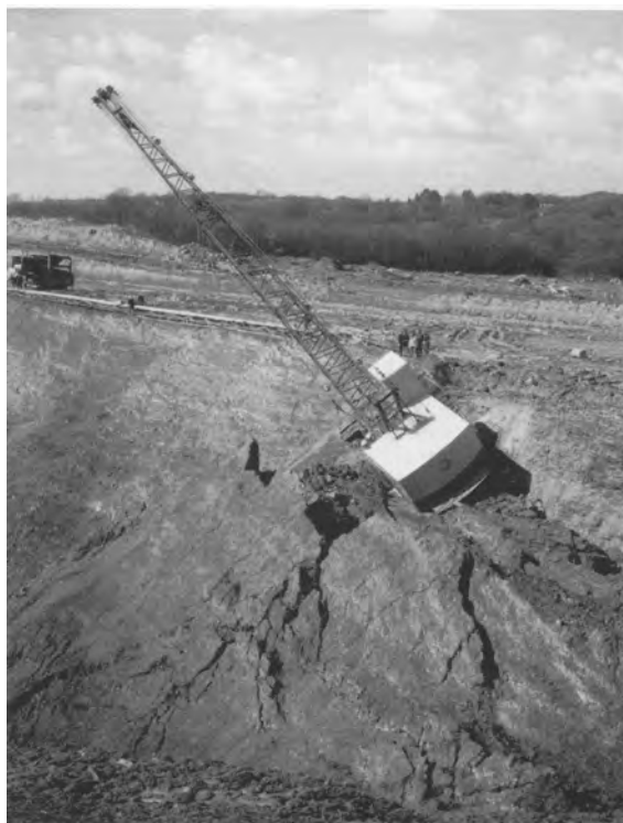
FIG. 7.1. Pit instability affecting production.
