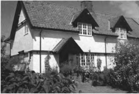
FIG. 13.9. Local authority housing built using claylump at East Harling, Norfolk, 1930.
