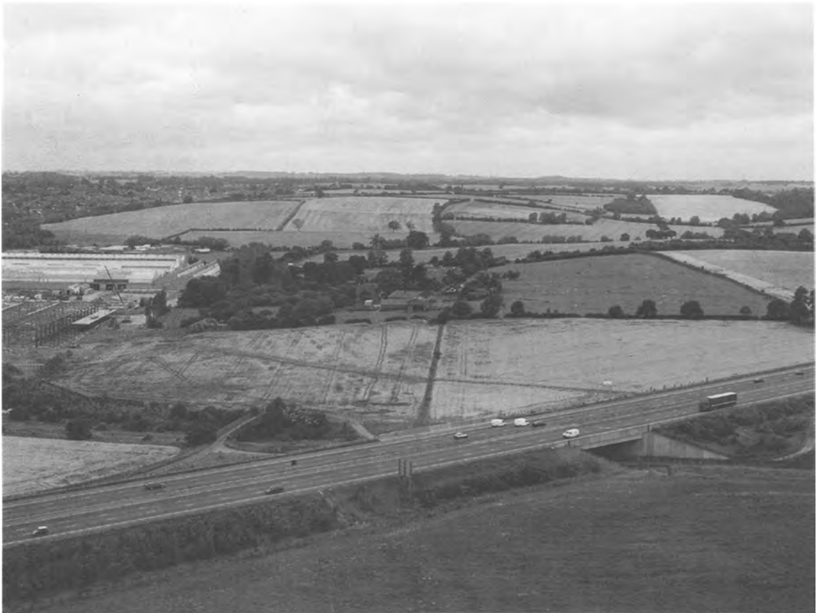
FIG. 10.1. (c) Highway embankment. Construction and design is to modern standards with adequate compaction and flatter slopes (Perry et al. 2003).
