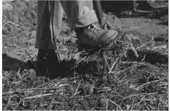
FIG. 13.3. University of Plymouth students demonstrating mixing for the cob building technique.
