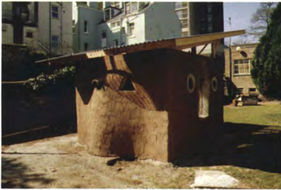
PLATE 14. Building erected at the annual cob building course at the CEA, University of Plymouth.
