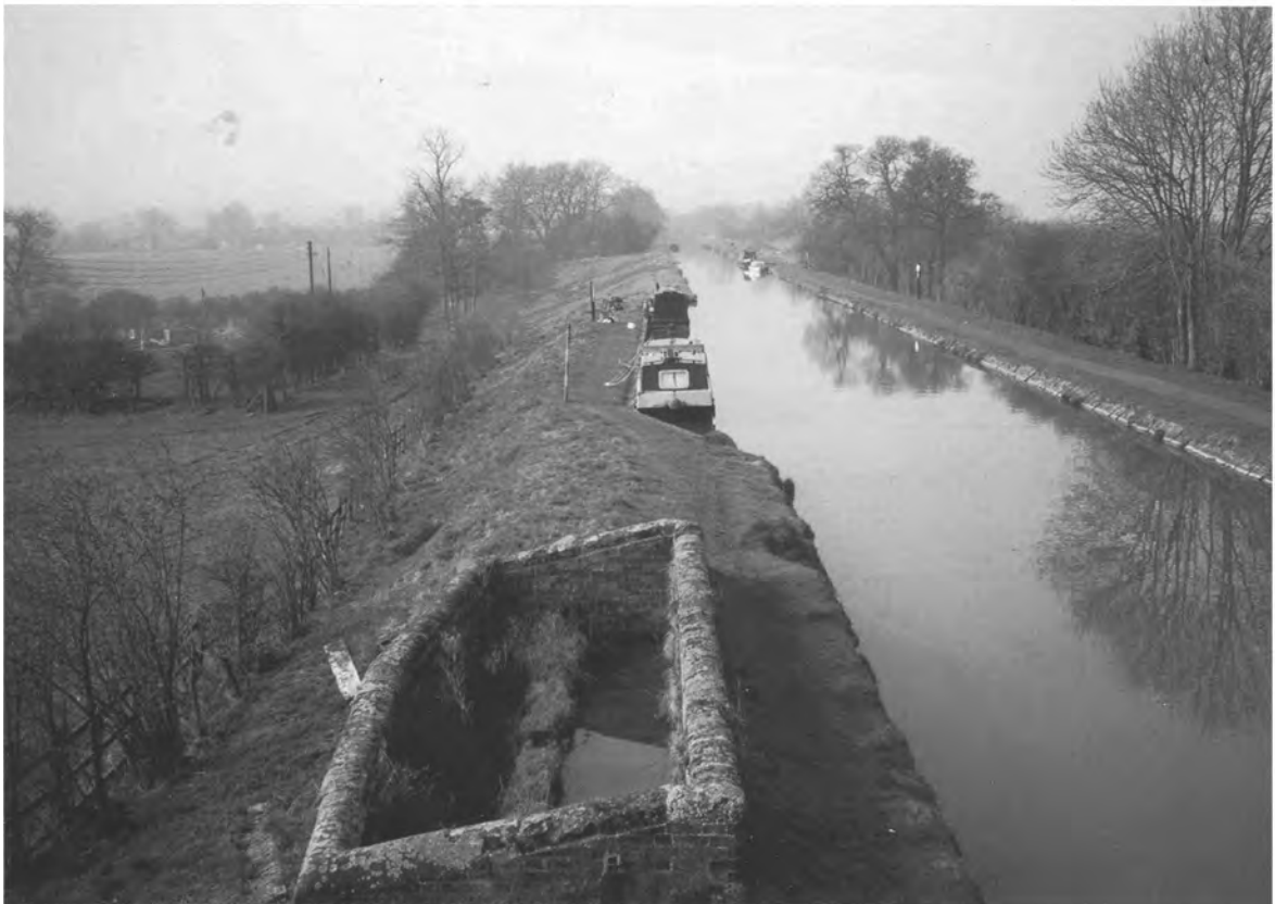
FIG. 10.1. (a) Canal embankment. Water is typically retained by a lining. Traditionally, puddle clay was used for this purpose, but replaced often utilised modern materials (Perry et al. 2003).
