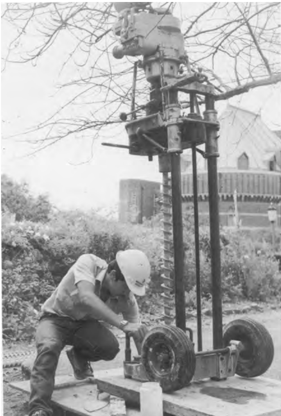
FIG. 7.10. Light probing equipment with a hollow stem auger.
