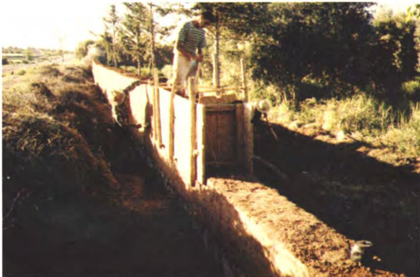
PLATE 6. Rammed earth being constructed in Morocco.
