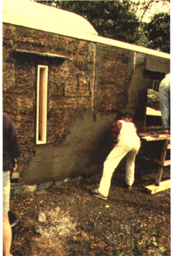
PLATE 7. Claystraw house under construction in Sweden by Helsinki University of Technology.
