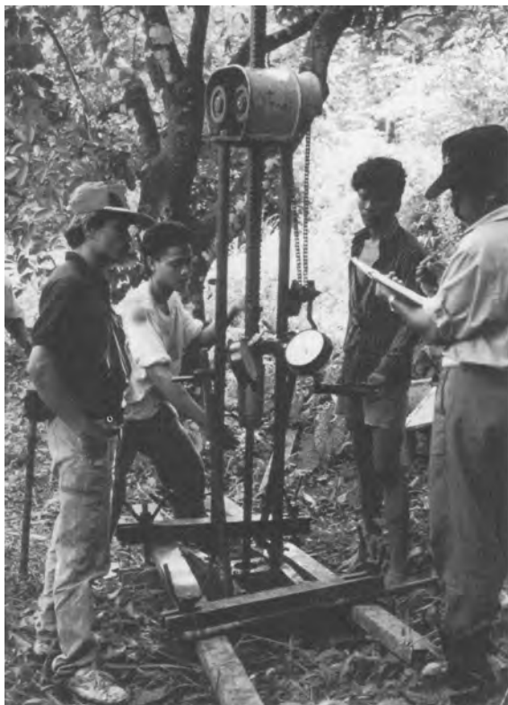
FIG. 7.13. Manually operated sounding rig.
