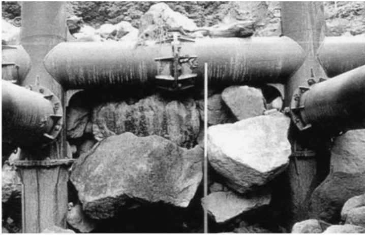
Photo 8.3 Clogging of a grid-type sabo dam.
