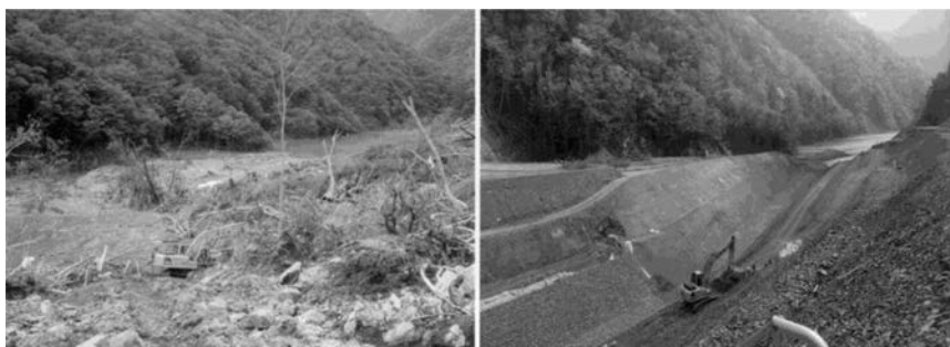
Photo 3.4 Before and after the emergency work for the Akadani landslide dam.
