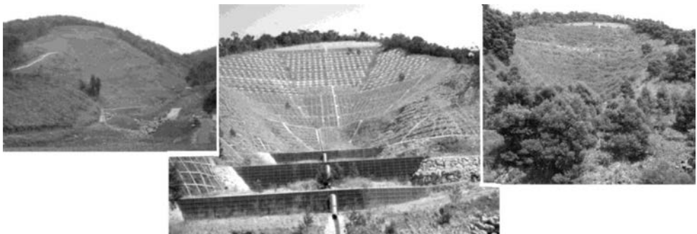
Photo 8.1 Hillside works on the landslide scar in the Harihara River basin.
