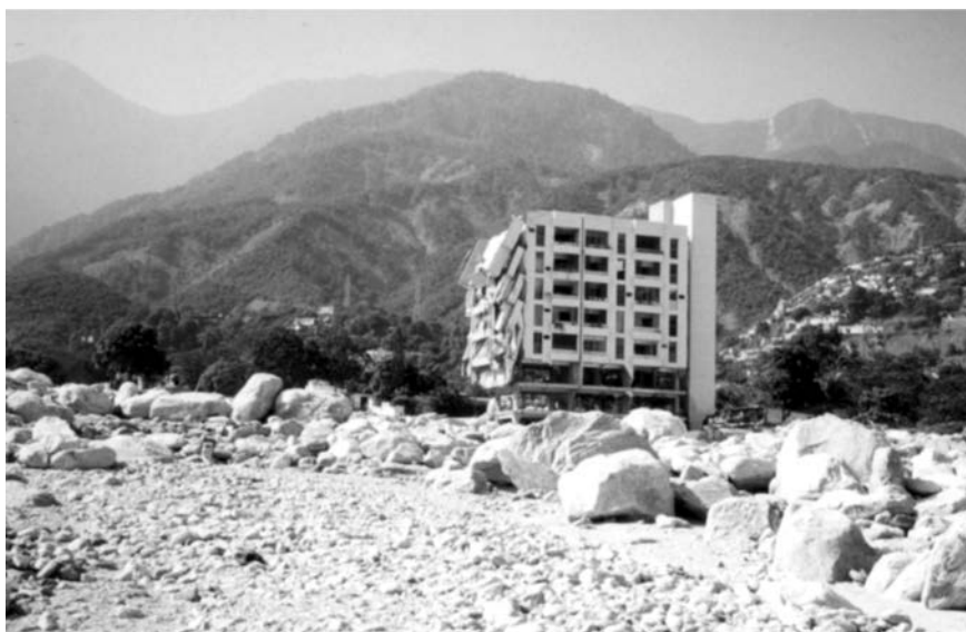
Photo 7.10 Building collapsed due to the direct strikes by boulders.
