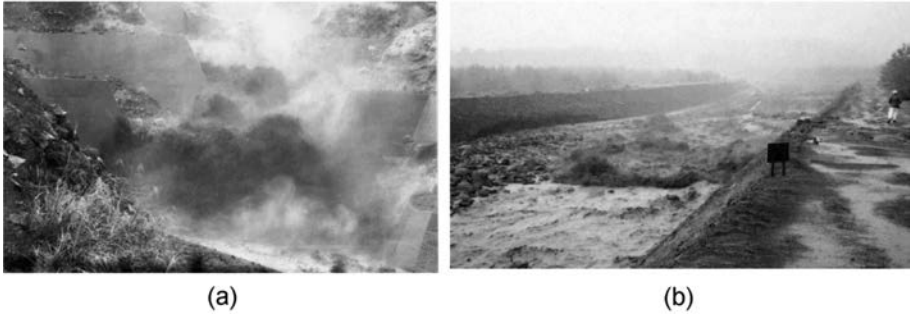
Photo 1.4 Debris flows in the Nojiri River, Sakurajima (Ohsumi Work Office 1988). (a) A debris flow passing through a sabo dam. 18 December 1986. (b) A debris flow flowing down the channel works.
