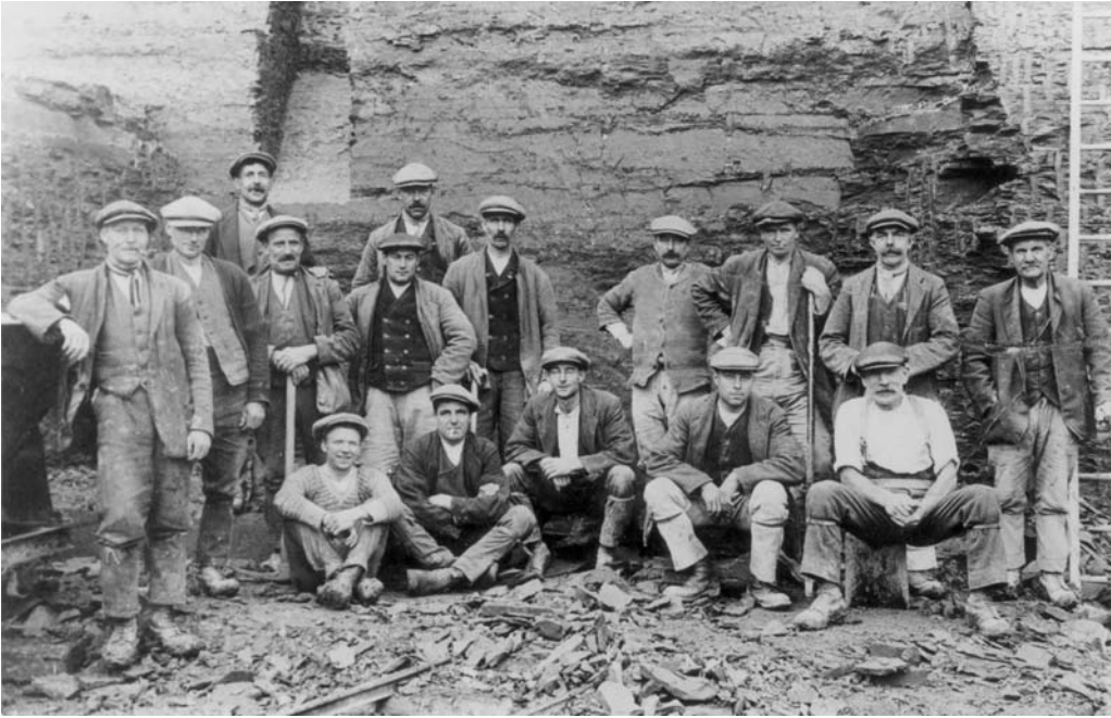
Fig. 5. ‘Clay getters’ in a Peterborough brick pit, date unknown but probably around 1900. Note the metal crowbars for hewing the clay by hand, and the chute in the background down which the clay from higher in the pit was sent into wagons on the pit floor. Photograph courtesy of and © Whittlesea Museum.
