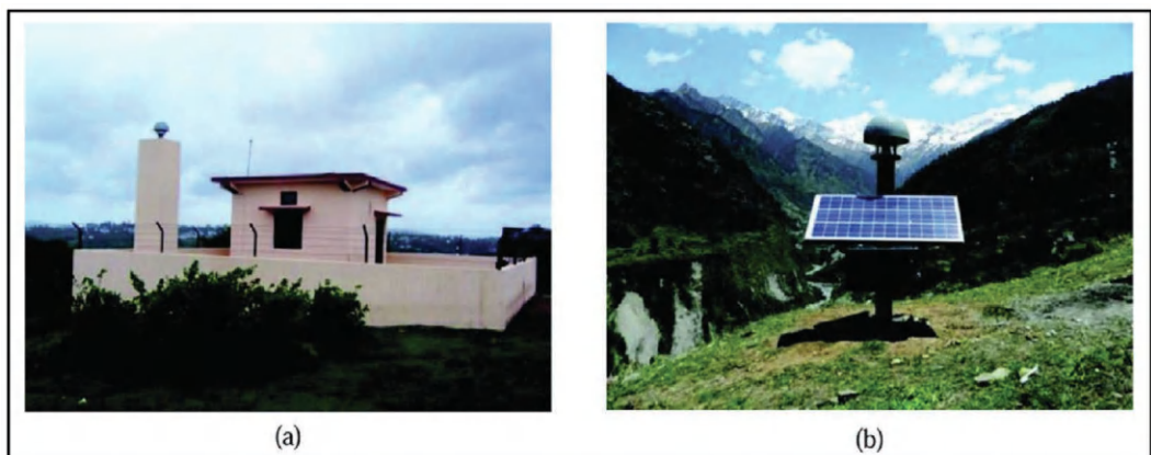
FIGURE 14.4 (a) A typical permanent GPS station at Port Blair, Andaman. (b) A typical semipermanent GPS station at Yamunotri in the Himalayan region.
