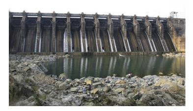
FIGURE 1.4 The "Maithon Dam", 48 km from Dhanbad coal belt town, India, is constructed on "Barakar River". The dam is 4,789 m long, 50 m high and over 65 km² water reservoir. It was specially designed, based on in situ rock competency and related structural features, for flood control and generate 60,000 kW hydroelectric power since 1957.
