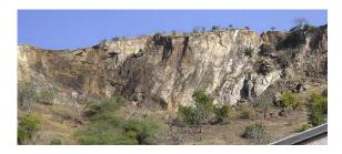
FIGURE 10.10 Surface subsidence over an operating underground zinc—lead open stope without any loss of man or material. The impact of the subsidence caused collapsing of crown pillars generating rich ore to draw without drilling and blasting costs.
