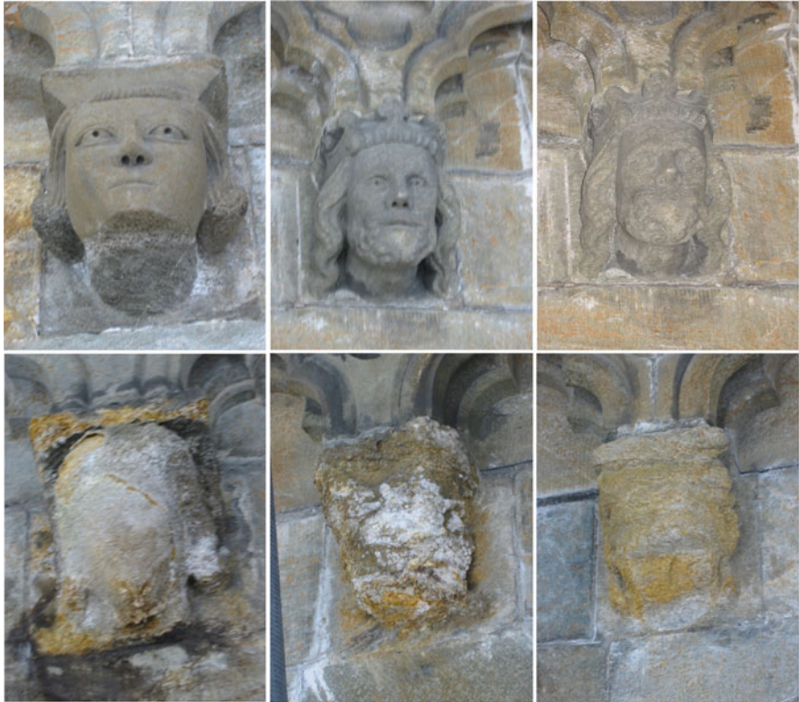
Fig. 12.21 Example of progressive stone decay at the Trondheim Cathedral, Norway (soapstone)
