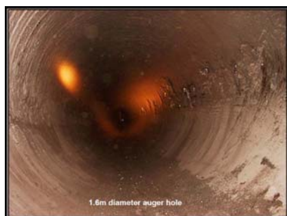
Figure 13. Hole 1.6 m diameter drilled by the augering machine UA 560 (left) and the view of heading side-wall after seam augering and holes sealing (right) (source: Buddery & Hill 2004).
