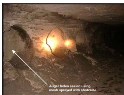
Figure 13. Hole 1.6 m diameter drilled by the augering machine UA 560 (left) and the view of heading side-wall after seam augering and holes sealing (right) (source: Buddery & Hill 2004).
