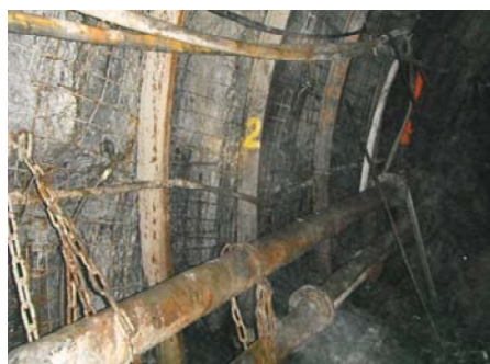
Figure 11. ŁPw mining supports installed in the riser 3 research on board the 504 in coal mine “Bobrek-Centrum” (Kuziak 2012).
