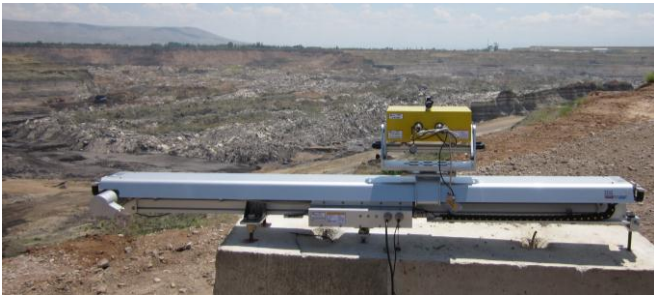
Figure 3. IBIS-M installation at Çollölar.
