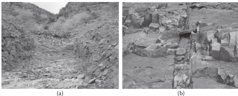
Figure 7.1 Rock foundation for a barrel aqueduct at 44.900 km of the Bansagar Feeder Channel, Sidhi District, Madhya Pradesh, India: (a) foundation trench and (b) rock condition at the founding level. (After Shukla, S.K., Allowable Load-Bearing Pressure for the Foundation of Barrel Aqueduct on Rock at km 44.900 of the Bansagar Feeder Channel, Dist. Sidhi, MP, India. A technical report dated 29 June 2007, Department of Civil Engineering, Institute of Technology, Banaras Hindu University, Varanasi, India, 2007.)
