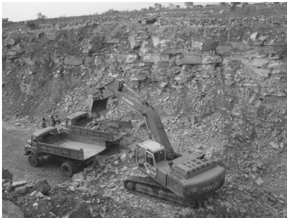
Figure 1.11 Heavily jointed rock mass at 0.080 km of the Meja-Jirgo link canal, the site for the construction of a canal head regulator, Mirzapur, Uttar Pradesh, India. (After Shukla, S.K., Allowable Bearing Pressure for the Foundation Rock/Soil at km 0.080 of the Meja-Jirgo Link Canal for the Proposed Construction of a Hydraulic Structure (Head Regulator), Mirzapur, UP, India. A technical report dated 11 June 2007, Department of Civil Engineering, Institute of Technology, Banaras Hindu University, Varanasi, India, 2007.)
