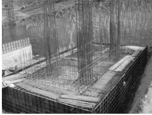
Figure 7.2 A raft foundation for an aqueduct under construction at 46.615 km of the Bansagar Feeder Channel, Sidhi District, Madhya Pradesh, India. (After Shukla, S.K., Allowable Load-Bearing Pressure for the Foundation of Aqueduct on Rock/Soil at km 46.615 of the Bansagar Feeder Channel, Dist. Sidhi, MP, India. A technical report dated 7 June 2006, Department of Civil Engineering, Institute of Technology, Banaras Hindu University, Varanasi, India, 2006.)
