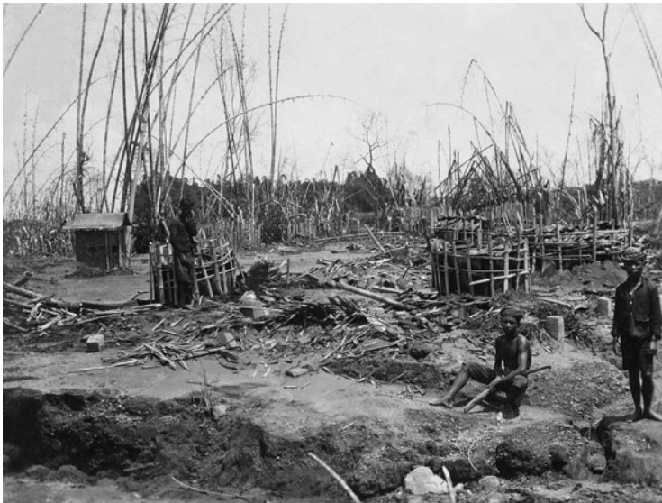
FIGURE 1.4 Photograph from 1931, surveying the destruction of Demong village from the Merapi eruption of 1930. Kroon verwoeste dessa Demong met graven en vliegenhuisje . Courtesy Balai Penyelidikan dan Pengembangan Teknologi Kebencanaan Geologi archive.
