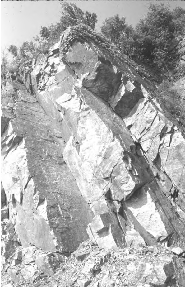
Figure 2 Rock highwall in rhyolite near Munsan, Republic of Korea, exhibiting three prominent joint sets of consequence to development of the site as a quarry. Such features should be taken into direct consideration in quarry dimensioning and in specification of the bearings of bounding highwalls; the horizontal width of the exposed joint faces is about 5 m, left to right. Photograph by the author.
