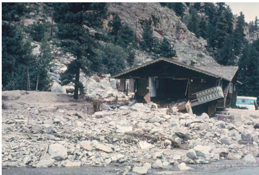
Figure 12 Results of an extreme flood in Big Thompson Canyon, Colorado, USA, in July 1976. Photograph by WC Bradley.
