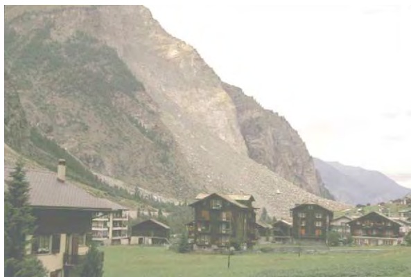
Figure 3 Large rockfall that occurred in the early 1990s in the village of Randa in the Pennine Alps of Switzerland.
