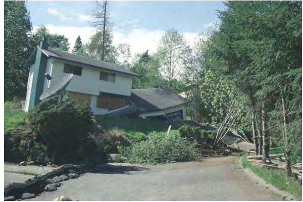
Figure 1 Home destroyed in 1998 in Kelso, Washington, by a thrust of soil under it as an ancient landslide reactivated, destroying 60 similar homes over a four month period. Note the main street in the foreground has also been destroyed.
