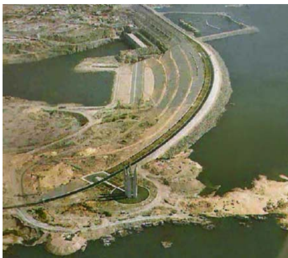
Fig. 70 The Aswan Dam ponding Lake Nasser in southern Egypt
