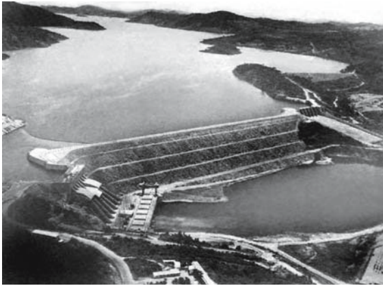
Fig. 89 The 113m high rock-fill dam at Akosombo in the Volta Gorge of southern Ghana, holding back an artificial lake of 8482 km 2 (1964)
