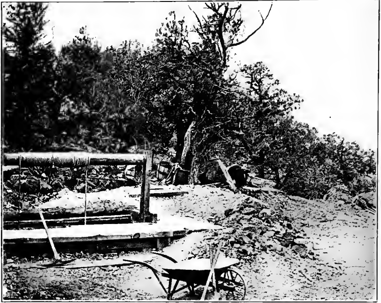
FIGURE 9. Shaft mining. Early method of raising quartz to the surface
