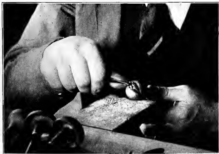
FIGURE 97. Bright cutting top and sides of prongs
