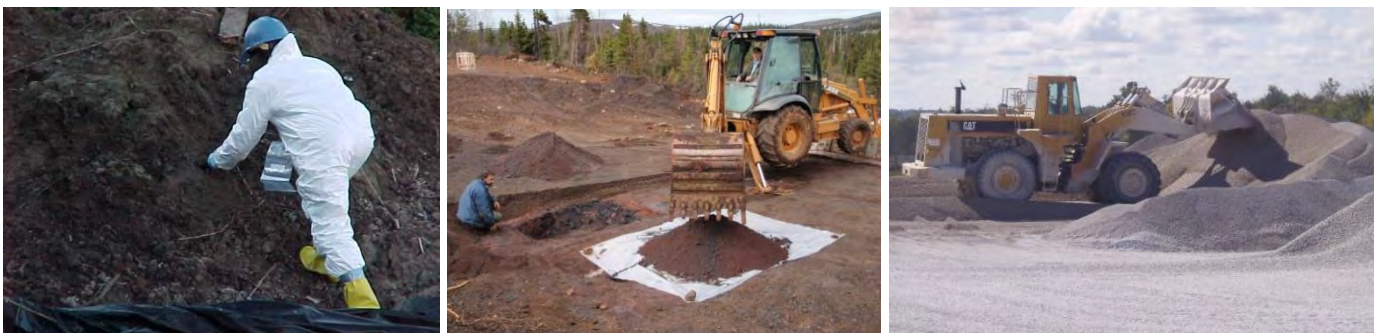
Figure 3.3: Three dimensional sampling on a stockpile means that the principle of correct sampling is violated (Source: (a) http://yosemite.epa.gov/R10/CLEANUP.NSF , (b) http://www.labradorironmines.ca/images/124m.jpg&imgrefurl (c) http://epg.modot.org/files/2/26/1001.jpg )
