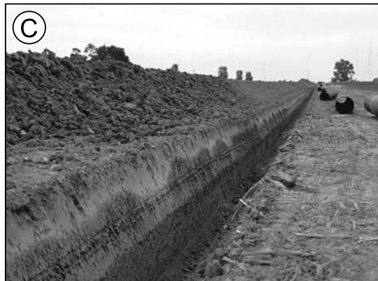
1 m lower than at the drill rig. Photo by L. R. Follmer. (c) Pipeline ditch in a Cisne–Newberry association in Fayette County, Illinois, showing the E horizon of the Cisne soil. Photo by L. R. Follmer.
