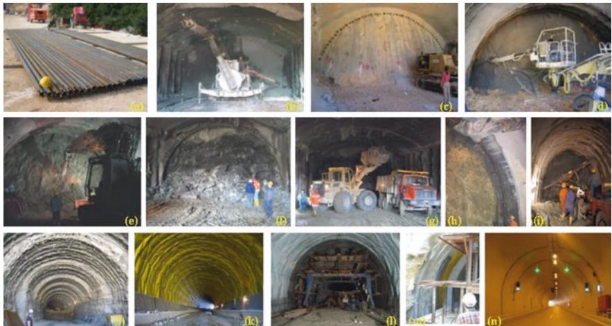
Fig. 21.10 Sequencing of tunnel construction at selected stages; (a) forepoles, (b) Installation of forepoles at tunnel face using forepoling machine, (c) view of tunnel face with forepole umbrella inserted, fiberglass dowels, and drainage pipes, (d) shotcrete being applied, (e) controlled excavation of face, (f) excavated material, (g) removal of excavated material, (h) installation of structural support—steel sets, (i) installation of further radial support—grouted rock bolts, (j) successive forepole umbrellas seen as well as bench, (k) installation of geomembrane, (l) installation of steel reinforcement for final lining, (m) detail of reinforced final lining, and (n) completed tunnel
