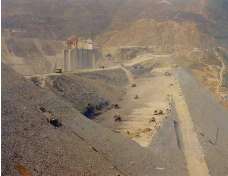
Fig. 25.7 TSQ.1 downstream view—zone III C progress in November 1998
