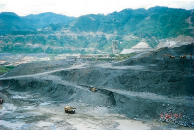
Fig. 25.9 TSQ.1 spillway approach channel entrance—mudstone excavation
