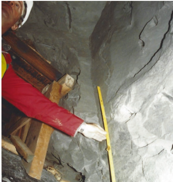
Fig. 18.8 Example of Q and Geotechnical log at well documented section for MRT/MST at ch. 22.526 m. Note that the most frequent ratio of J_w/J_r is 6/1, but 9/1 is also frequent. Refer to Fig. 18.9 example linking overbreak to J_w/J_r .
