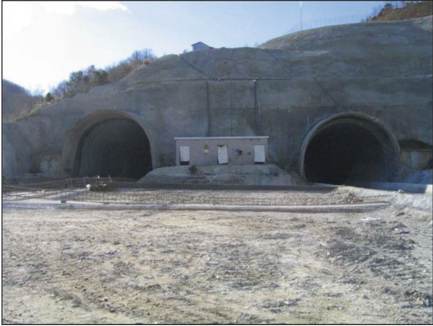
Fig. 21.17 Driskos Northern Portals during construction in 2003
