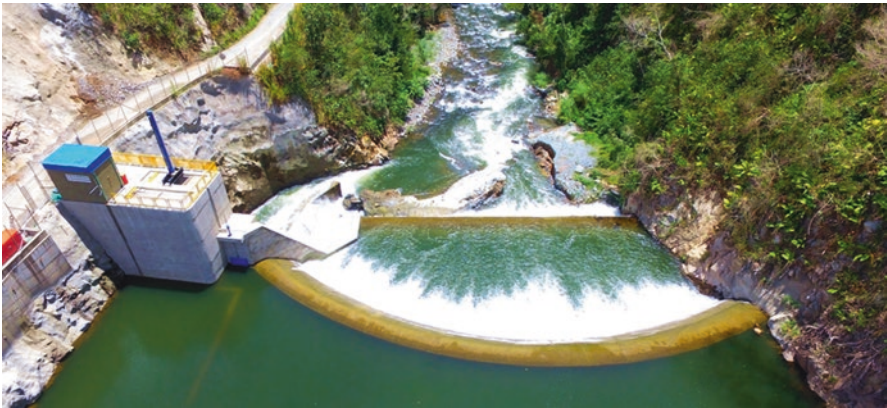
Fig. 24.5 Drone view of the completed dam under operation
