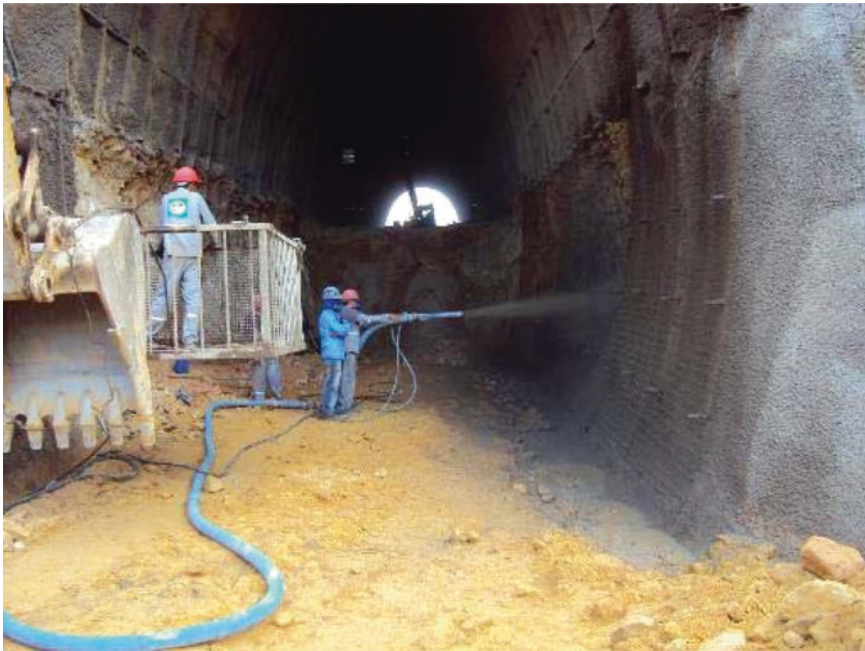
Fig. 5.18 Application of shotcrete and steel grid in bench walls (Photo E.L. Pastore)
