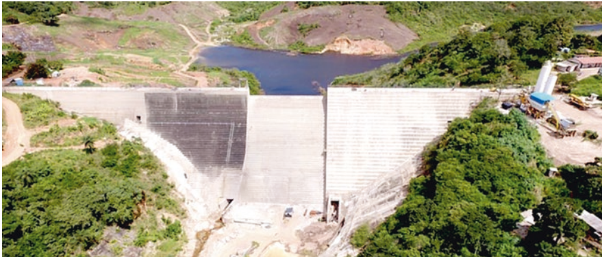
Fig. 24.17 Camará Dam after complete refurbishment
