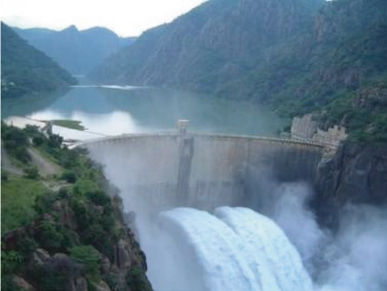
Fig. 20.16 Cahora Bassa dam (HCB 2018)
