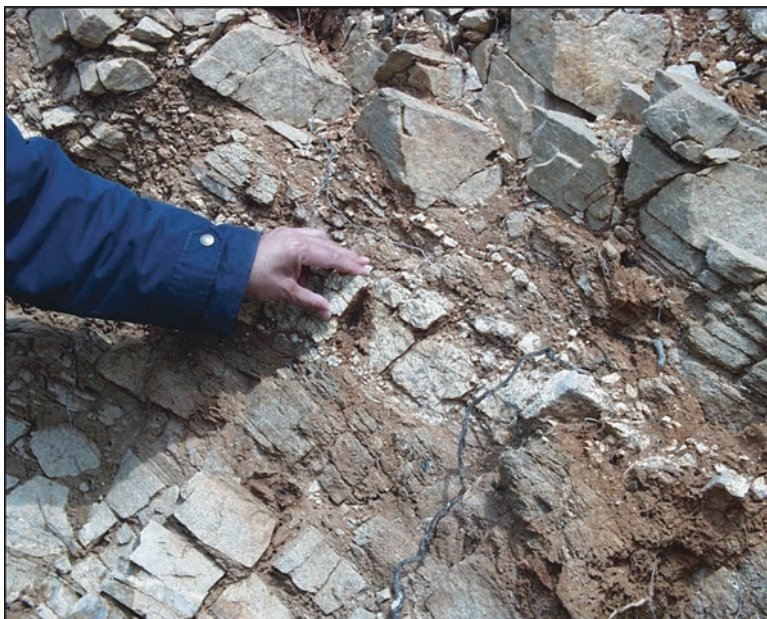
Fig. 19.14 Intense weathering along the gneissic bands but also along intersecting joints
