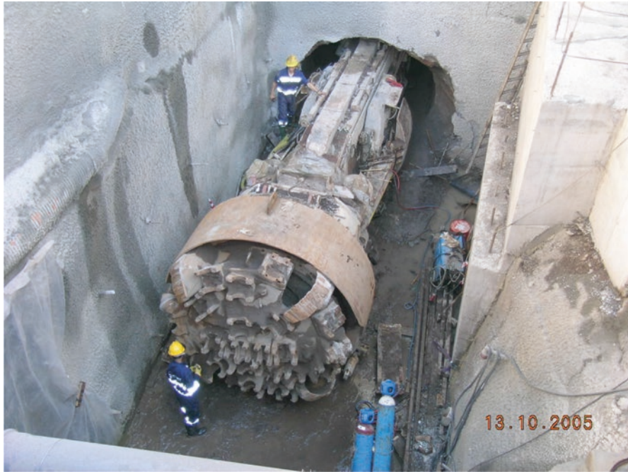
Fig. 20.4 TBM used at Covão tunnel
