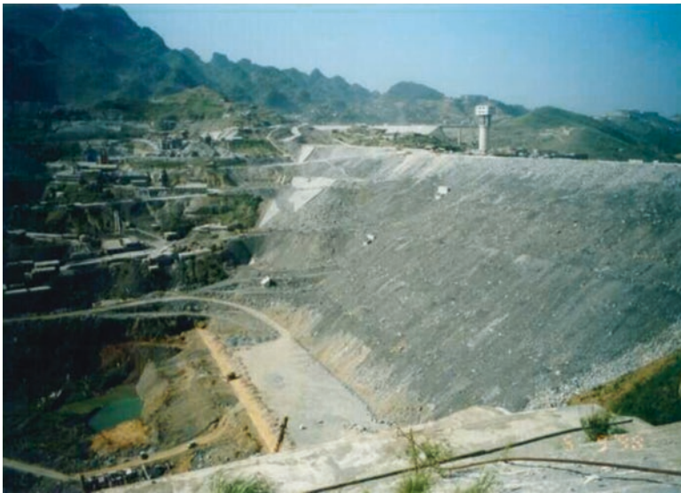
Fig. 25.6 TSQ.1 downstream view in August 1998. Detail of slope of zone III C of “mudstone”
