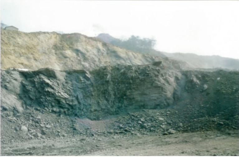
Fig. 25.8 TSQ.1 “mudstone” excavation borrow areas
