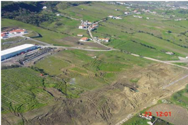
Fig. 4.24 Aerial view of the unstable area
