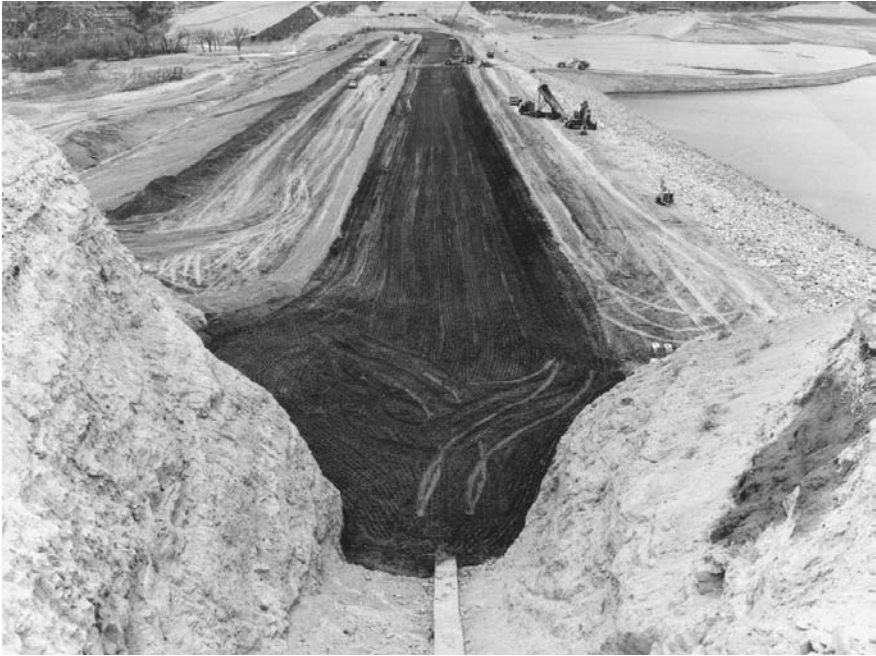
FIGURE 14.12 Embankment compaction, Greyrock Dam, Greyrock, Wyoming.
