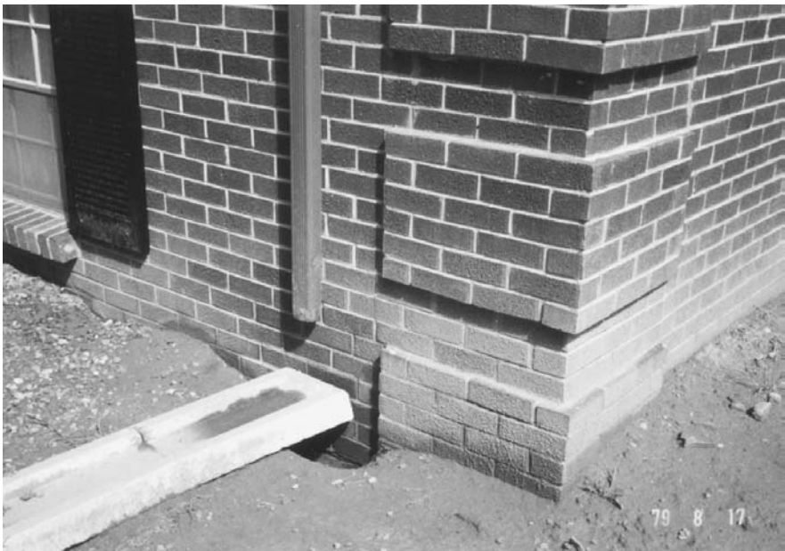
FIGURE 13.9 Down spout drain into backfill.
