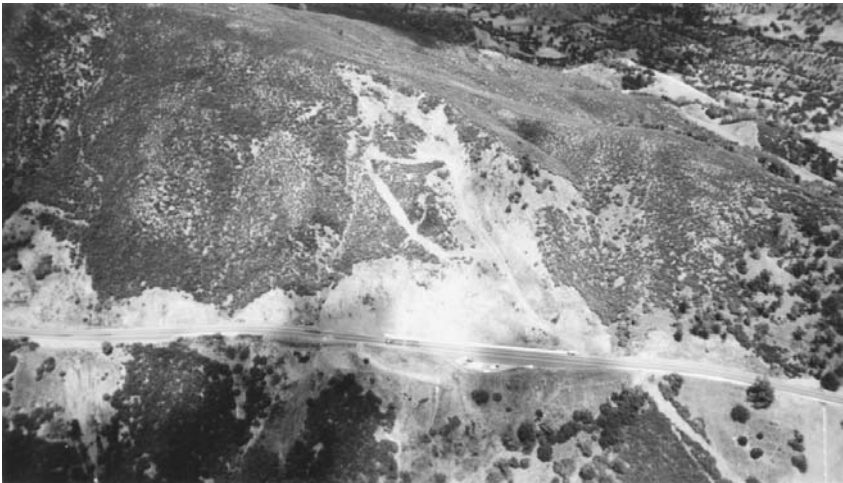
FIGURE 14.10 Typical landslide along a highway cut area.
