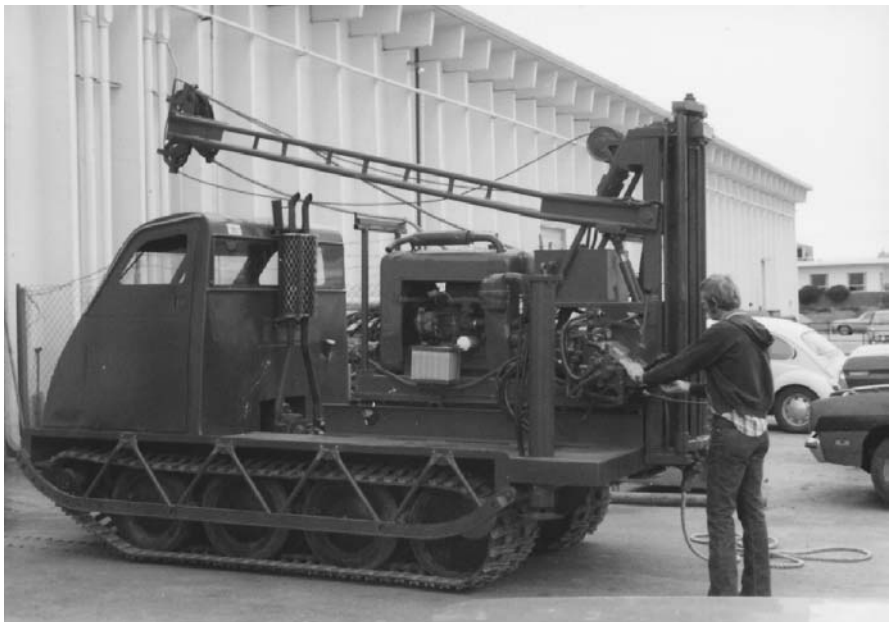
FIGURE 2.3 Tractor-mounted auger drilling rig.
