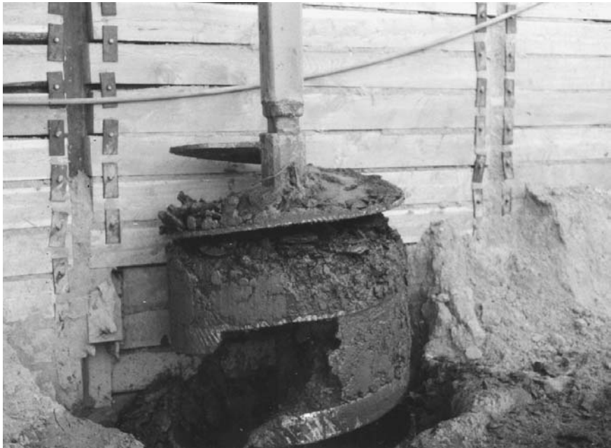
FIGURE 10.3 Large-diameter pier drilling for a high-rise building.
