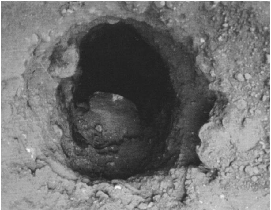
FIGURE 17.1 Boulder in the drilled pier hole.
