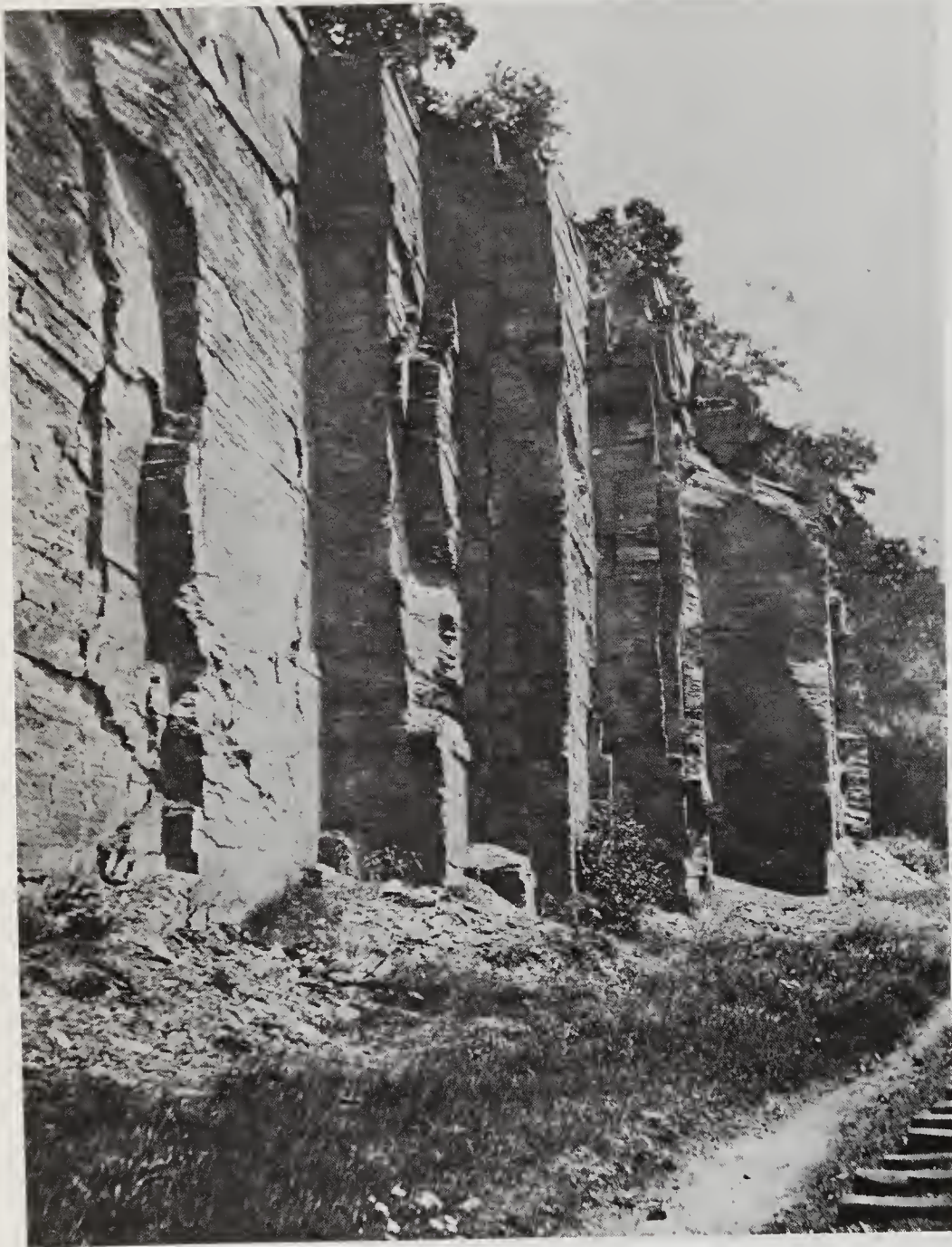
Plate 16. Joints. Vertical joint planes in Portage Formation. Tompkins County, New York. Photo: E. M. Kindle, U. S. Geological Survey.
