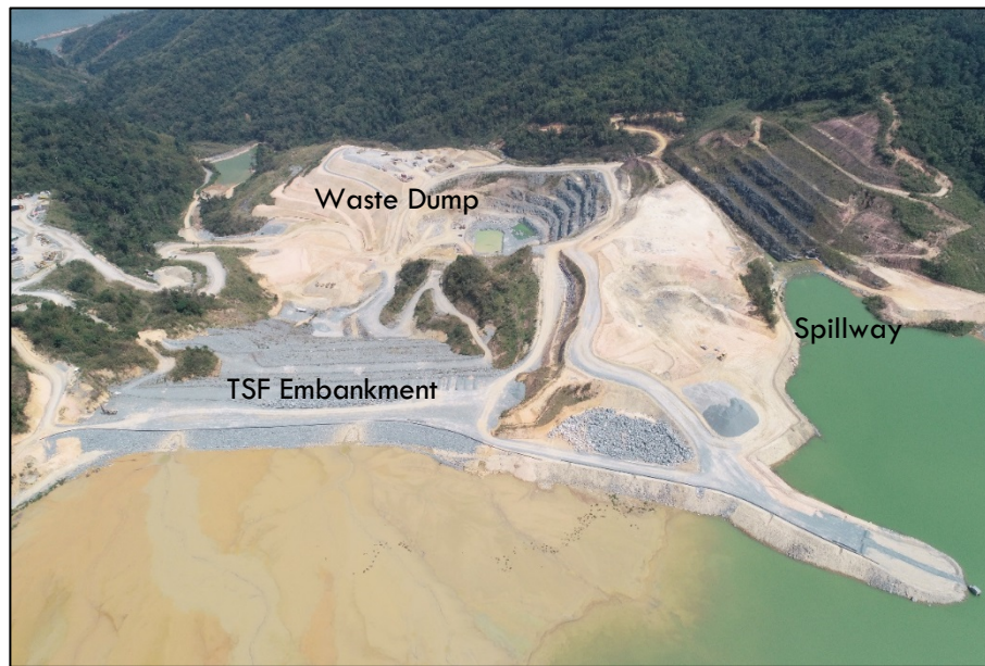
Figure 5: Ban Houayxai tailing storage facility embankment and spillway
