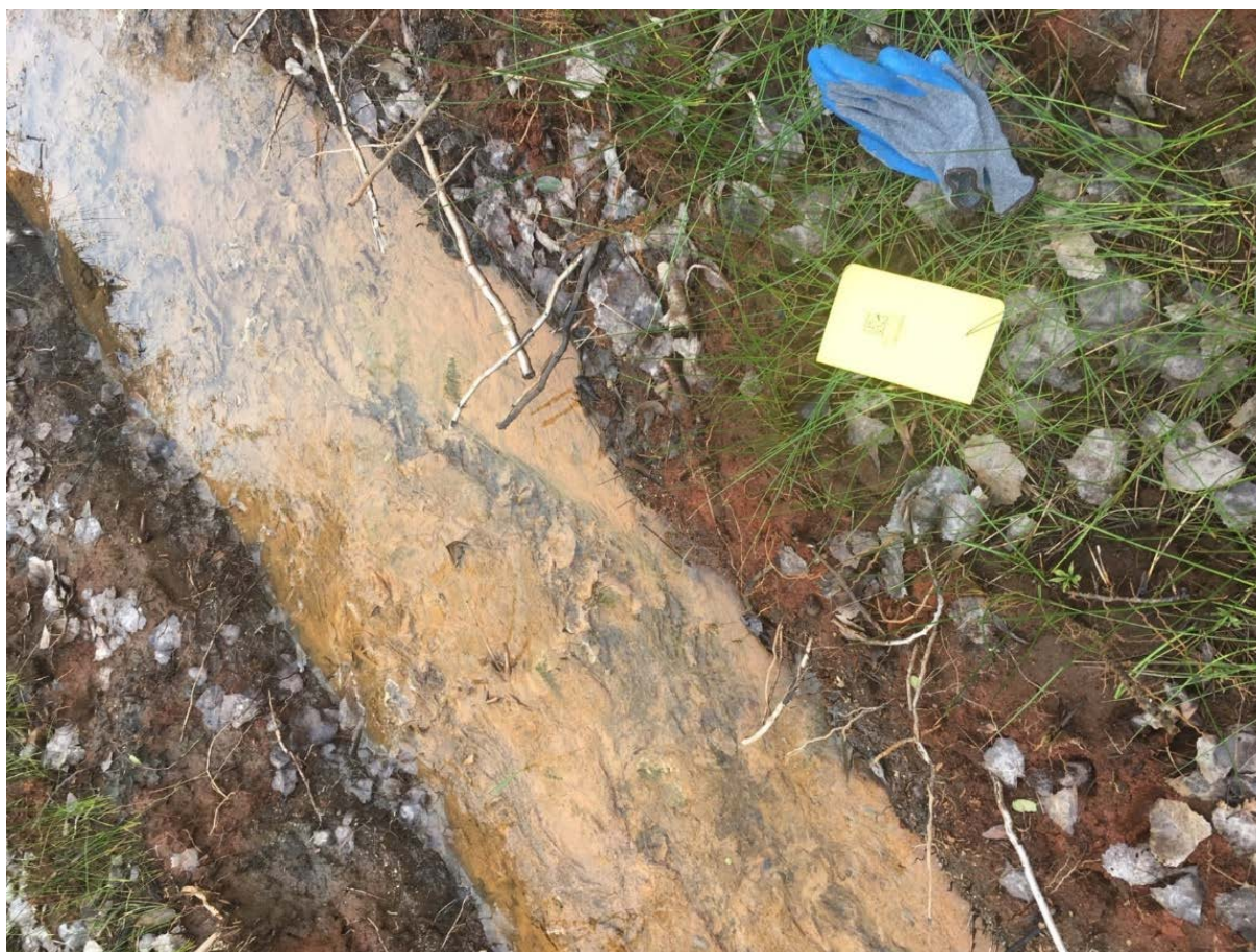
Figure 3: Iron hydroxide precipitation in tailing dam drainage channel
