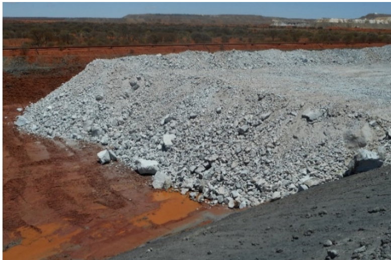
Figure 7: Waste rock buttress along the downstream slope of the CDTSF internal embankment
