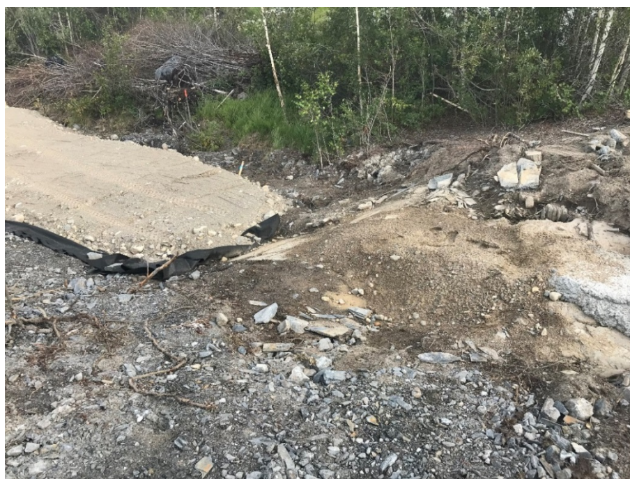
Figure 6: Placement of sand-bentonite mixture on prepared foundation of BGM liner key trench
