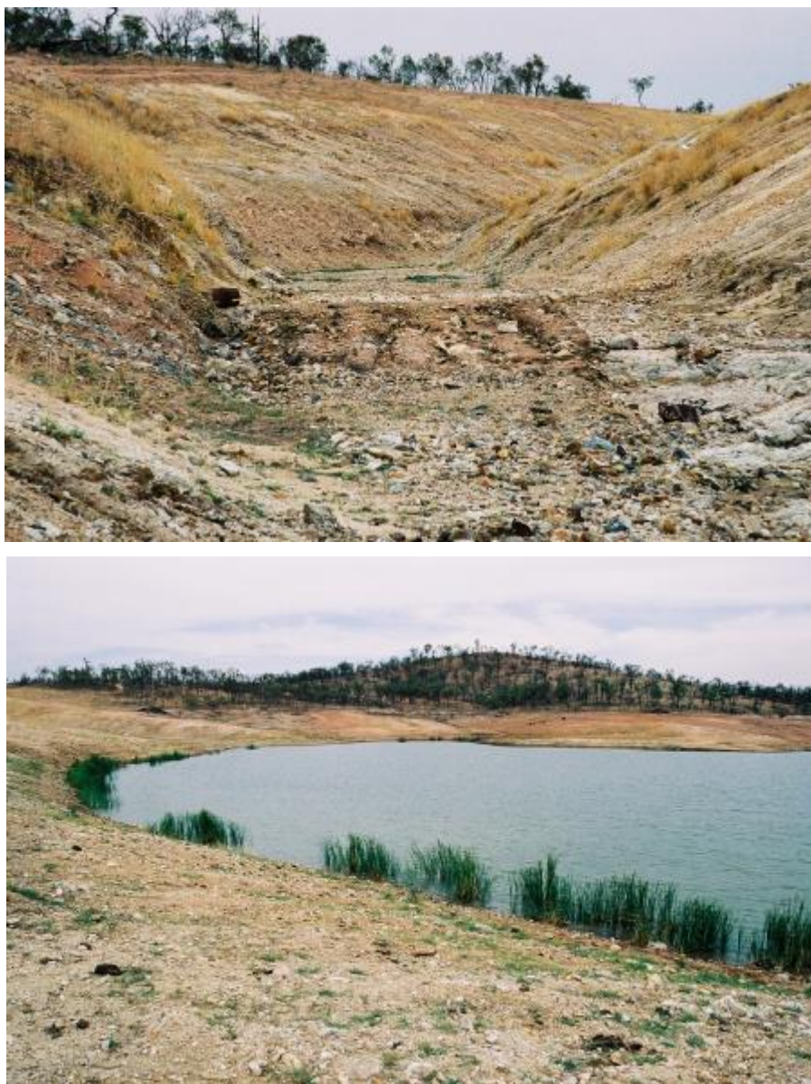
Figure 7: Tailings dam closure: (above) spillway cut through natural rock, and (below) lined sediment pond located just upstream of spillway
