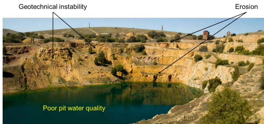
Figure 1: Open pit geotechnical and erosional instability and poor pit water quality
