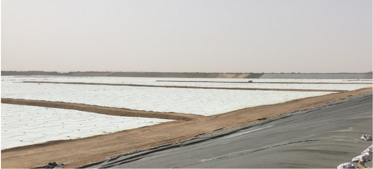
Figure 6: Liner ballast access roads within the TSF basin
