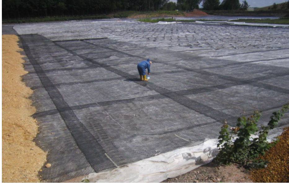
Figure 4: Geogrid T-shape installation
