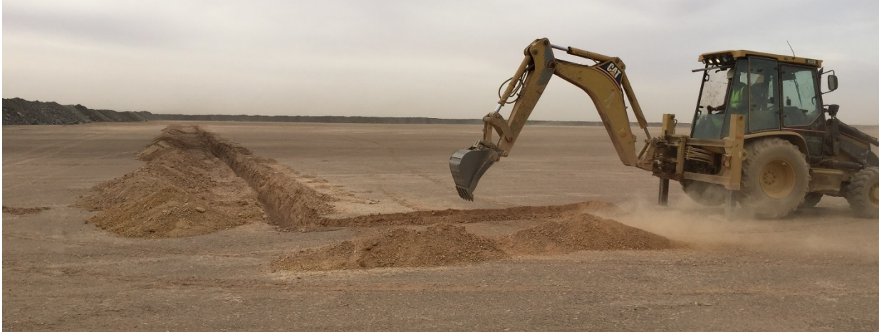
Figure 5: Construction of temporary anchor trench in basin of TSF for liner installation, upstream embankment slope not yet formed
