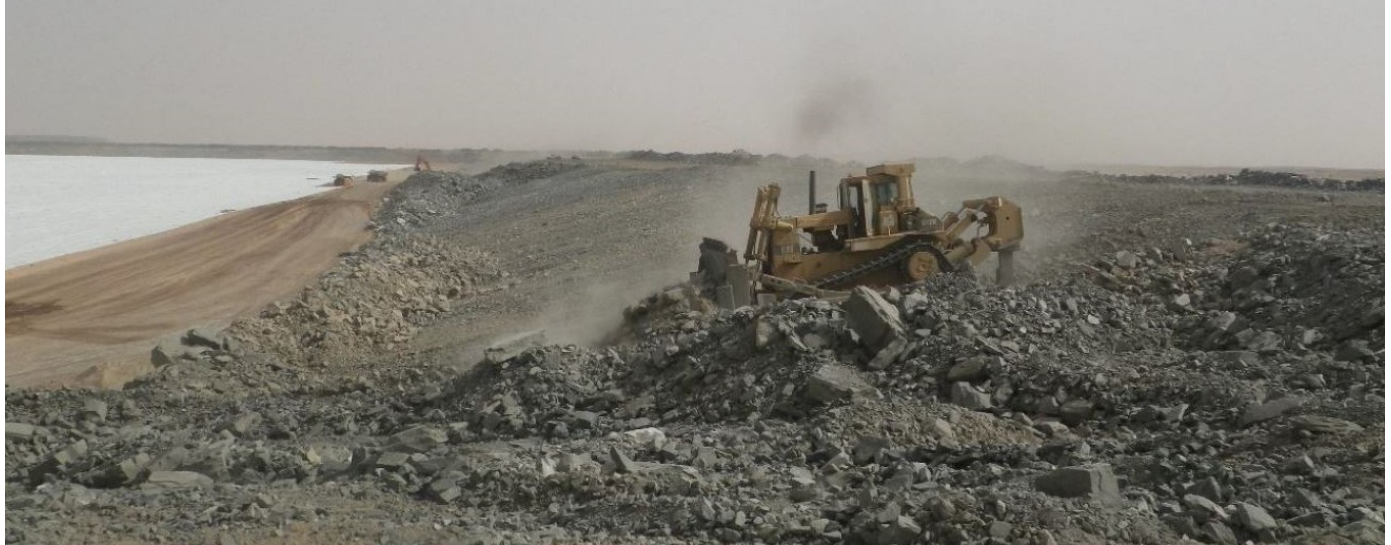
Figure 2: Forming of upstream slope
