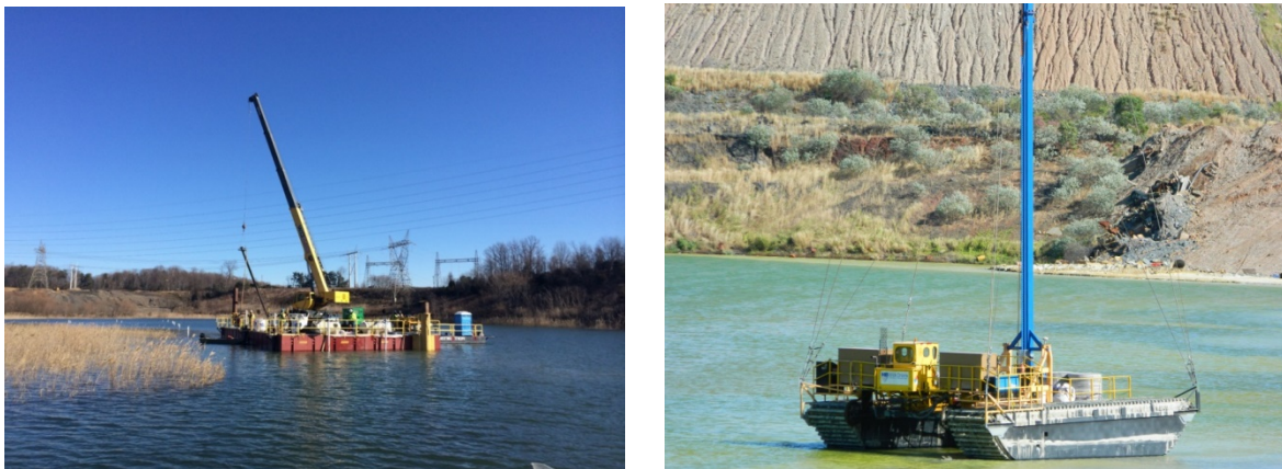
Figure 4: Wellpoint installation from floating barge (left). Wick drain installation from customized pontoon (right)
