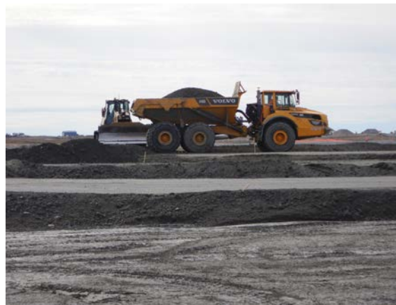
Figure 8: Tailings placement, spreading, and compaction
