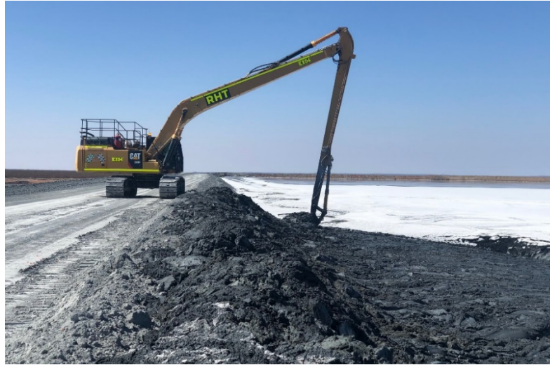
Figure 6: Tailing excavation and stockpiling along upstream toe of the internal embankment
