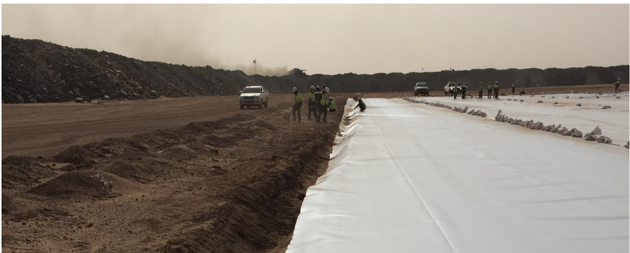
Figure 7: Proximity of waste rock placement to geomembrane installation (note the dust generation)
