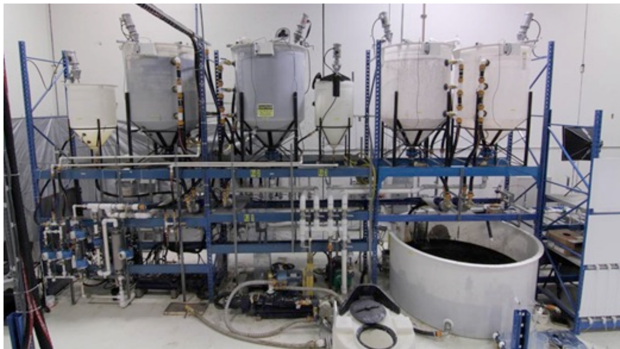
Figure 1: Flocculation facility primary piping and tank support frame
