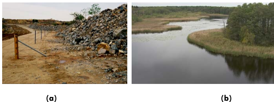
Figure 2: Post-closure treatment of open pits: (a) bunding and fencing, and (b) backfilling and pit lake
