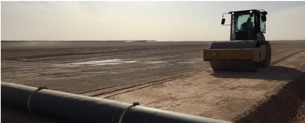
Figure 4: Smooth rolling of the foundation immediately before geomembrane placement (rough grading by dozer in background)
