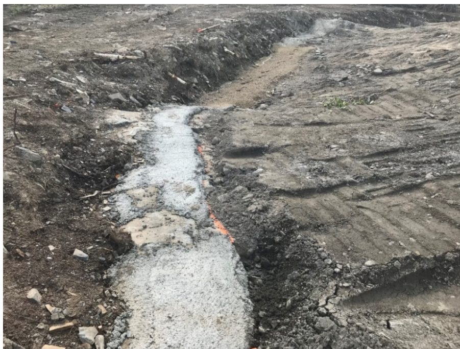
Figure 5: Preparation of bedrock surface in a key trench
