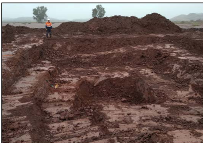
Figure 3: Battered excavation in tailings, enabling recovery of block samples and a large volume of disturbed material
