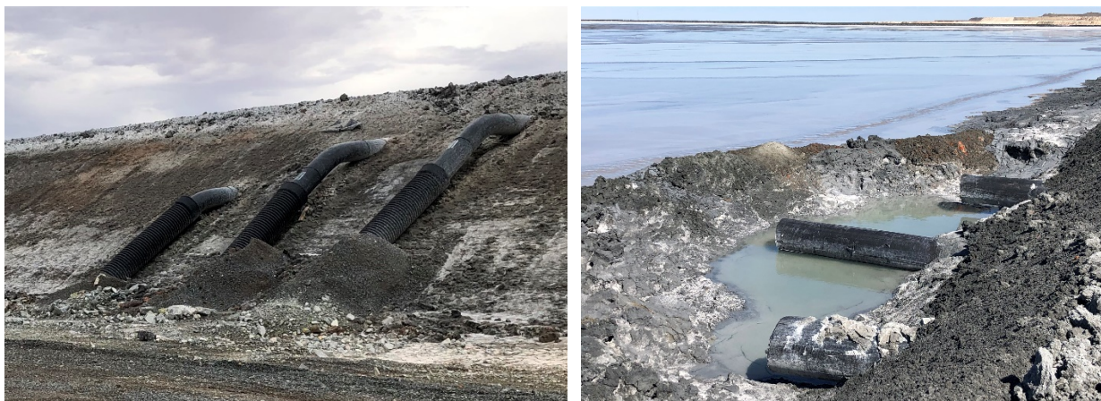
Figure 5: Decant pipe arrangement along the downstream slope (left) and at the inlet (right)
