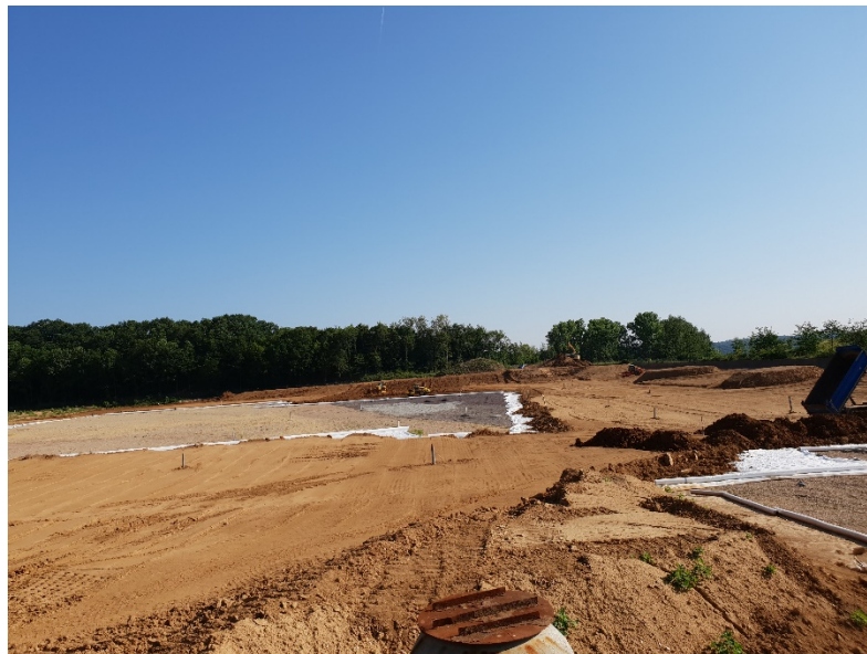
Figure 6: Installation of the top soil
