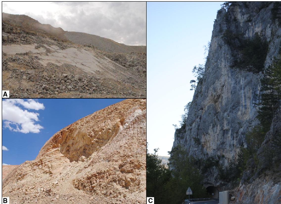
Fig. 10 a Plane failure in quartzite bench (slope height = 12 m) from a large opencast mine in Western Australia. b Wedge failure in sandstone (slope height = 30 m). c Stable limestone slope in Serbia (slope height = 70 m)
