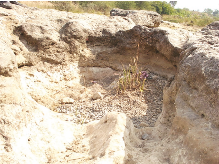
Plate 5.2a Photograph showing accumulation of gravel deposits in low lying area
