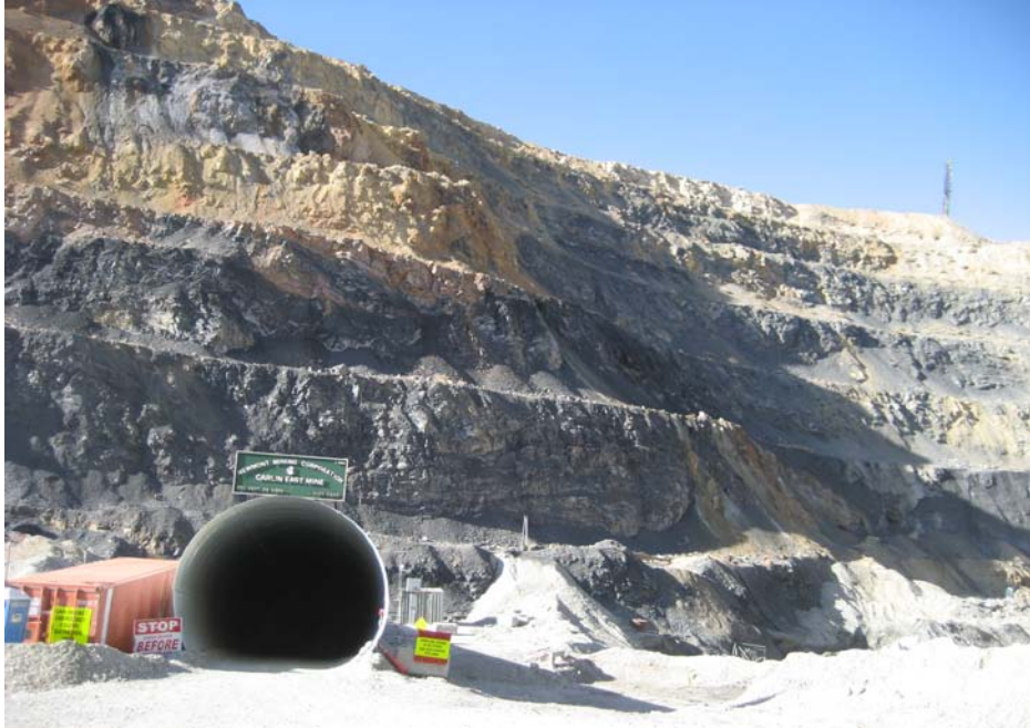
Blast-hole drill (upper right) at the Carlin mine, near the portal of the Carlin East underground mine.
