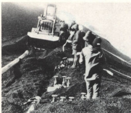
On May 4, 1973, workmen laid additional pipes to carry seawater up onto the lava flow front and tephra bulwark to cool and harden the still-flowing lava behind the chilled lava margin.
