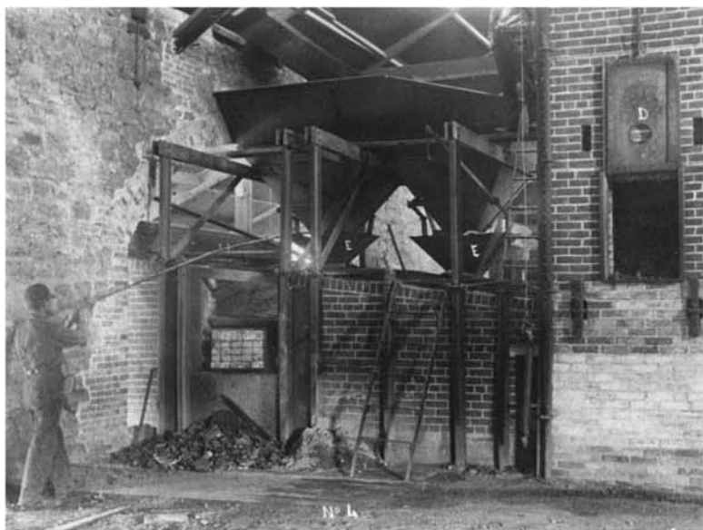
Charging a furnace at the Argo smelter. Jesse D. Hale, photographer. Colorado Historical Society, Denver.
